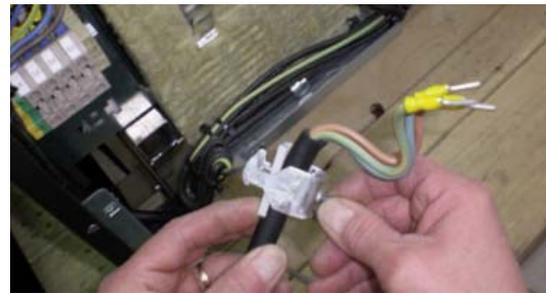
4. Insert the strain relief device into the hole and push it to the left. Tight up the power cord and strain relief device with the screw.
