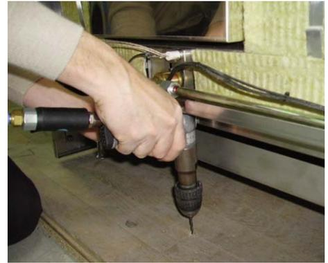
4. Where the floor consists of tiles, concrete or another hard material, drill a 10 mm diameter hole, push in the plug and screw the stud into it.
