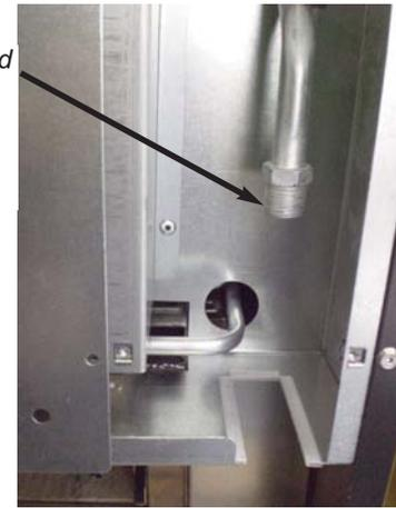
Connect flexible metal appliance connector to the adapter on the range. Position range to permit connection at the shut-off valve.
